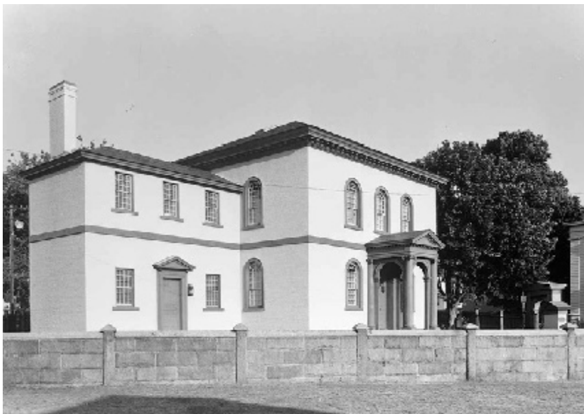
Touro Synagogue, Rhode Island Touro Synagogue, designed by Peter Harrison, constructed in 1762. Photograph by Jack Boucher, 1971. Library of Congress.
