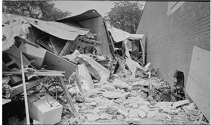
Bomb damage at the Gaston Motel
