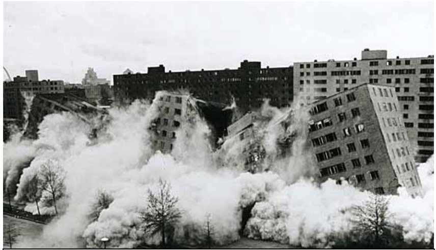
Demolition of the Pruitt-Igoe projects in St. Louis
